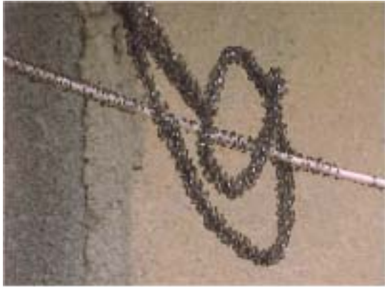
(A) Rusty wire
