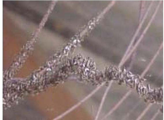
(A) Rusty wire
