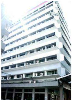
Chamlong Harinasuta Building
