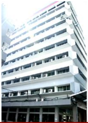
Chamlong Harinasuta Building
