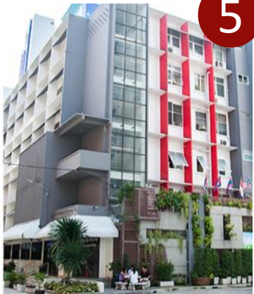
Sornchai Looareesuan Building
